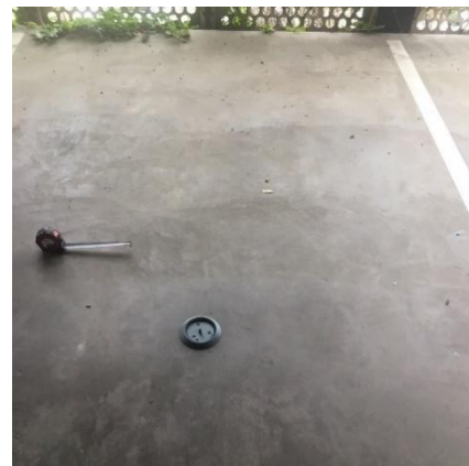
Figure 9 Sensor base installed
