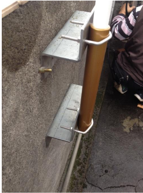
Figure 27 Customized Metal Bracket – Image 3
