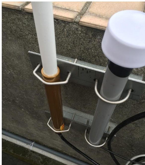
Figure 26 Customized Metal Bracket – Image 2
