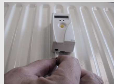
7-15 INSERTING THE SEAL
