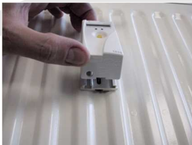
7-14 MOUNTING EURISII ON HEAT CONDUCTOR
