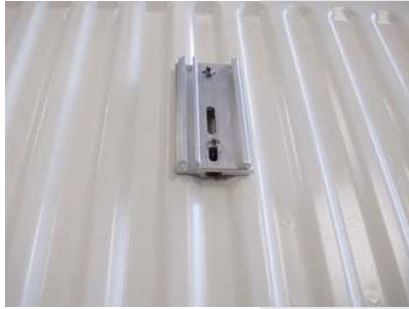
7-11 MOUNTING OF HEAT CONDUCTOR
