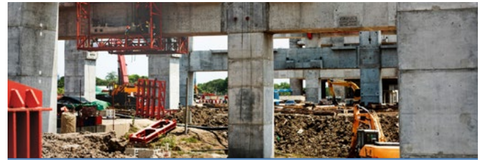
CONSTRUCTION SITE INVENTORY
