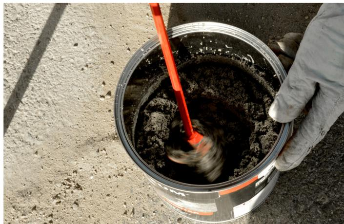
*Figure : Preparing the Epoxy resin mixture*
