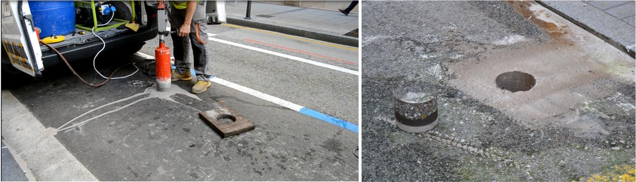
Figure : Making a hole in the pavement
