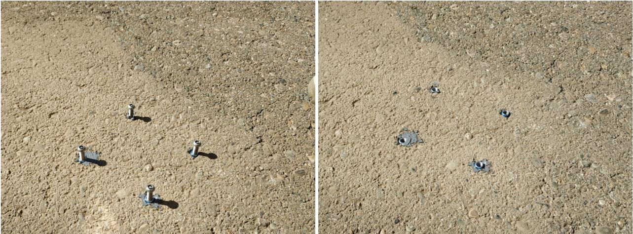
Figure : Final anchor installation (step 7)
