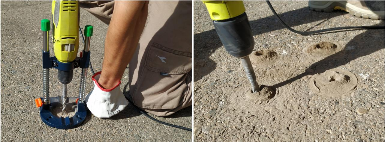
Figure : Drill the holes (step 1)
