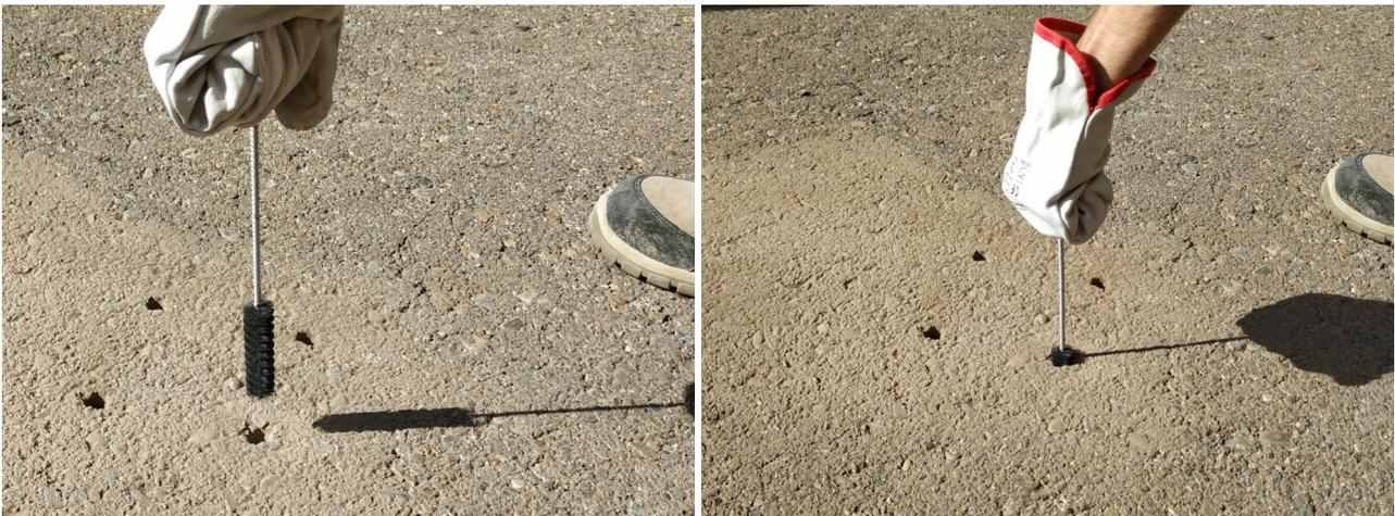
Figure : Brush the hole (step 3)
