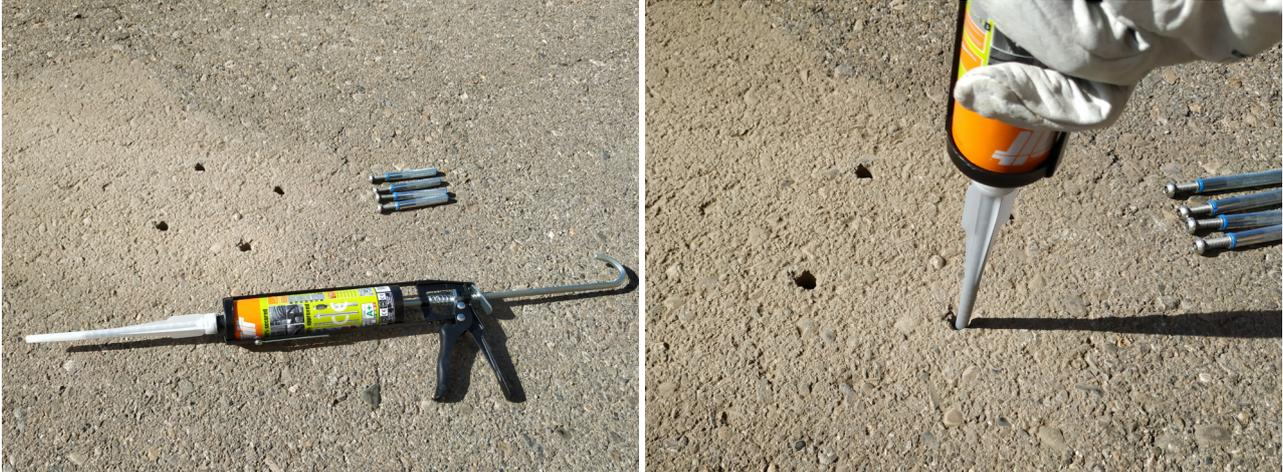
Figure : Inject chemical fixing adhesive (step 5)
