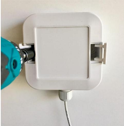
Ensure that the cable gland is fully tightened. Open the hatches on the front of the casing and drill two screws into the wall.
