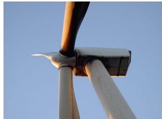
Wind turbine leaking oil. © Copyright Neil Owen
