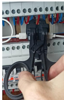
Fig. 12 – tag-Plyers used to position a watTag
