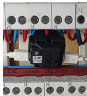
Fig. 5 – watTag_S installed
