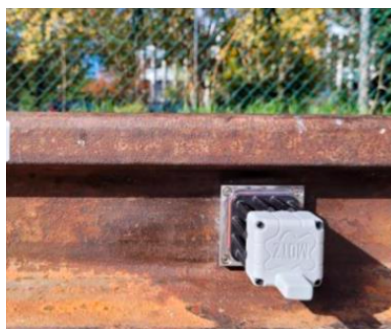
Railway tracks temperature monitoring
