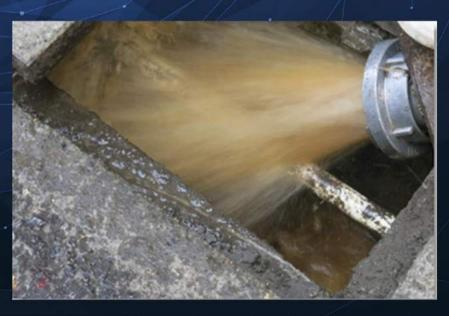
Automatic purge is a method of circulating the water in a network and to avoid stagnation on branches that are not very stressed, a source of contamination by the time of exposure to the various deposits that are bacterial vectors.
