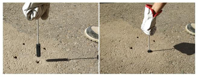
Figure: Brush the hole (step 3)
