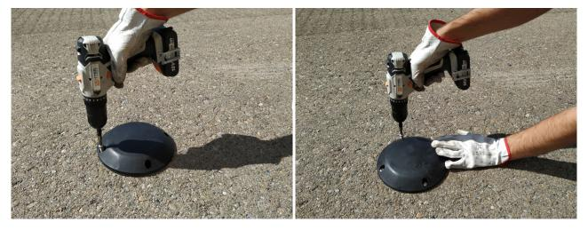
Figure : Screw the node
