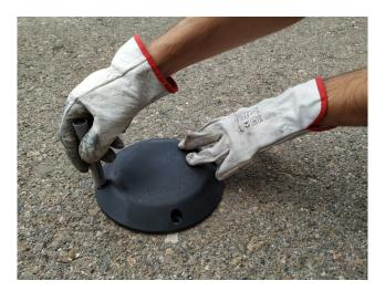
Figure : Marking the holes for the node
