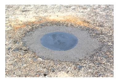
Figure: Final Epoxy application
