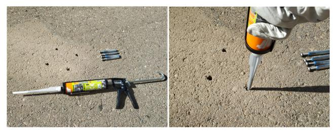
Figure: Inject chemical fixing adhesive (step 5)
