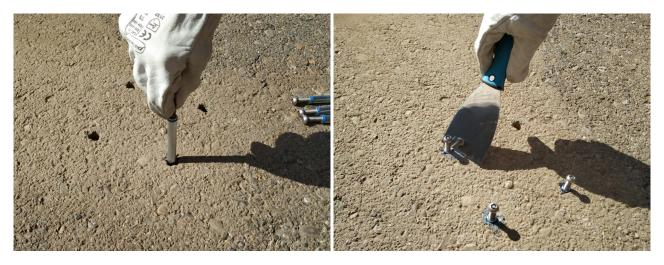
Figure : Insert the anchors (step 6)
