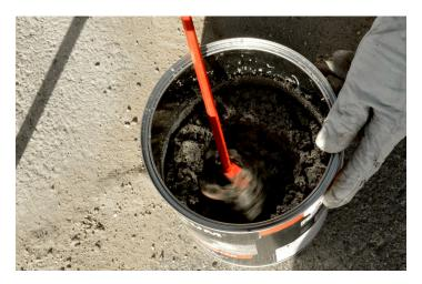
Figure: Preparing the Epoxy resin mixture
